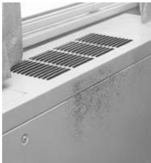
Mold growing on the surface of a unit ventilator. Moisture control is the key to mold control. If items are kept dry, mold does not grow.
