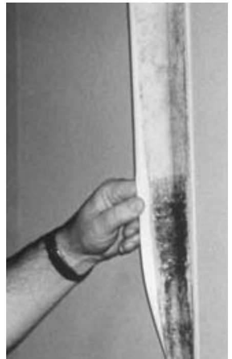
Mold growing on the back side of wallpaper. If you believe that you may have a hidden mold problem, consider hiring an experienced professional. (Photo courtesy of Environmental Protection Agency.)
